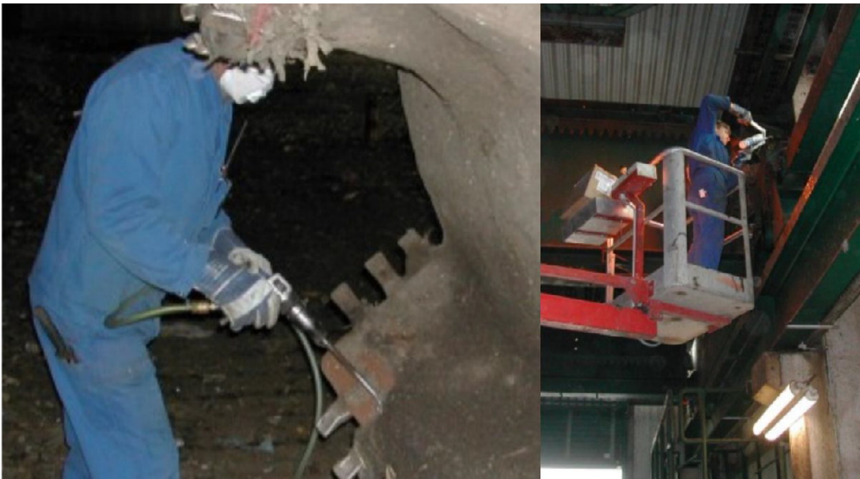
Fig. 4 Example: Maintenance of the equipment
