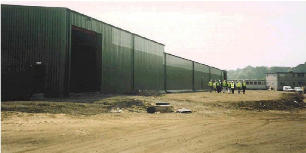
Fig. 1 Treatment facility in Wimborne
