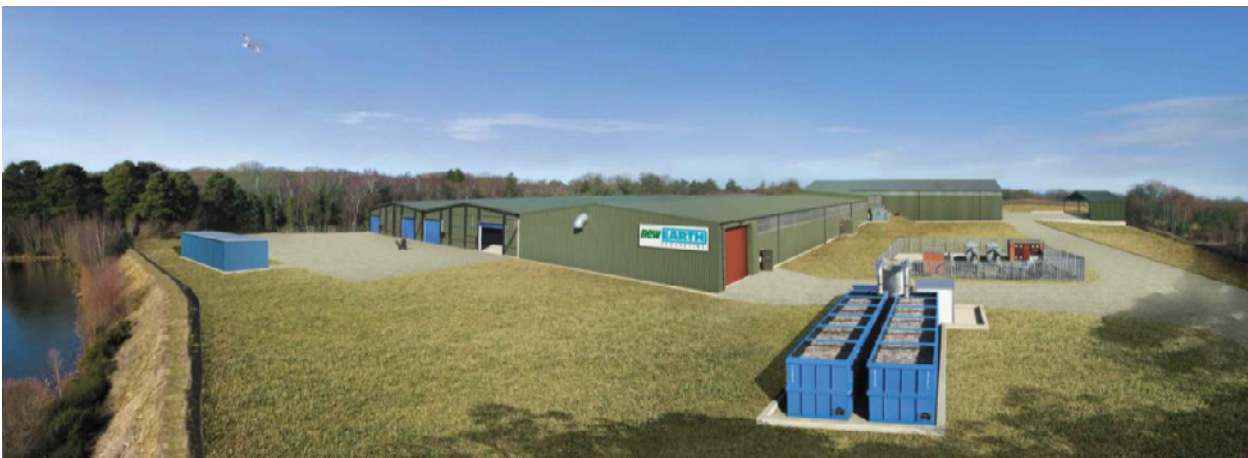
Fig. 16 Wimborne treatment facility
